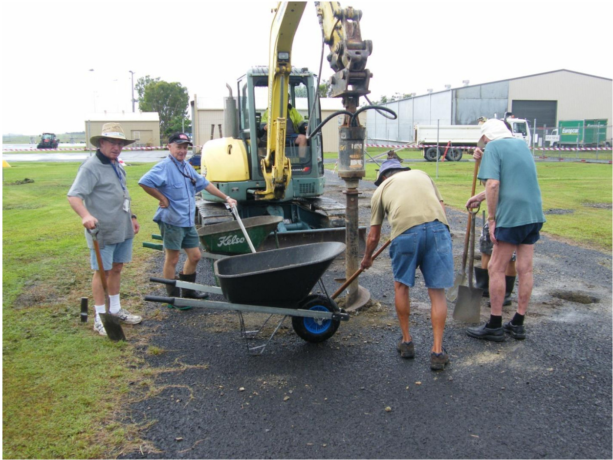
Figure 2 Boring holes for foundations
